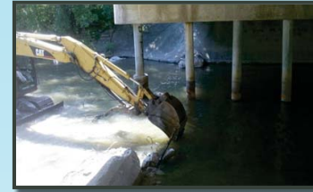
Removal of the dam sill.
