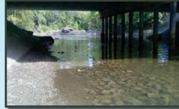
The rock for the riffle was placed under the bridge. A 6" thick layer of smaller stone was placed first and overtopped by larger rock.
