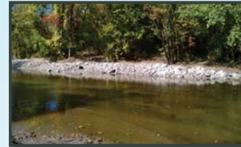
With the construction of the north bankfull bench, two storm sewer extensions and outlets were installed.
