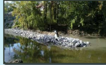
Storm pipe was installed at existing outfall to extend the pipe through the proposed bankfull bench to the stream channel.
