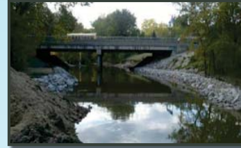
Sand bankfill was placed behind the stone toe. Geotextile fabric was used between the stone toe and the sand backfill.
