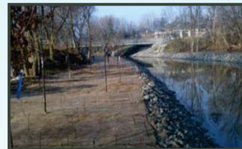
With tree planting complete, seed was placed and erosion control blanket was installed on the bankfull benches. Then, live stakes were installed.
