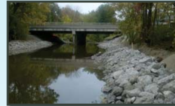
Bankfull bench construction view looking upstream towards bridge
