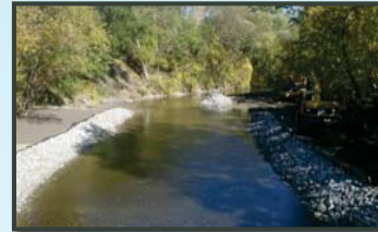
Work continued on the bankfull benches downstream of the bridge
