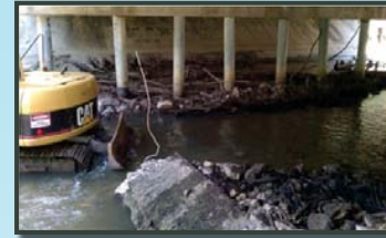
Lowering of water level at the dam by notching the dam.
