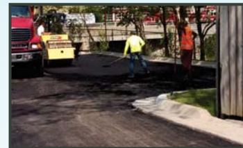
Replacing parking lot.
