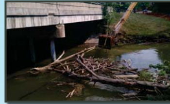
Removal of log jams.
