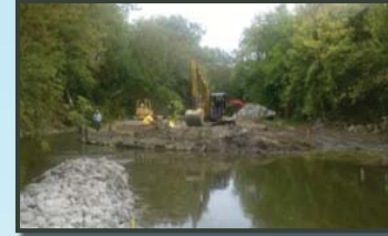
A portion of the existing island was excavated. It was eventually completely removed.
